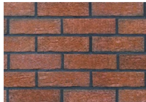
Tower bridge (HF09)
